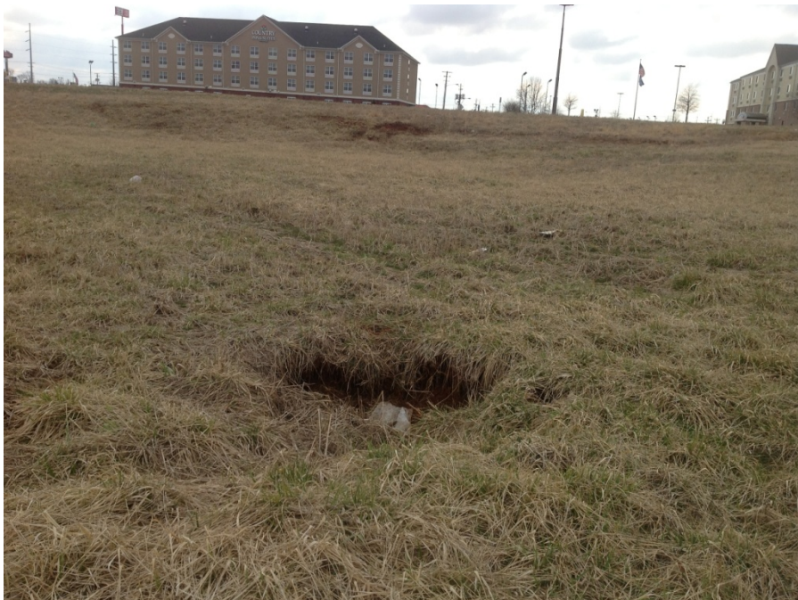
Open throat in the area of the Ken Dale Boulevard to Wall Street connector
